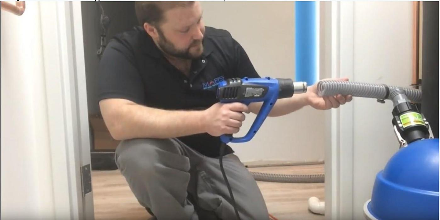
**Step 4** – When the hose is soft, slide it over the barbed fitting and tighten the hose clamp.
